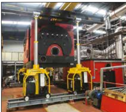
▼ Moving and positioning a 25 ton boiler using the ML40 Mini-Lift Gantry.
